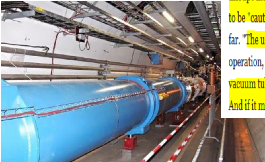
Tunnel of the Large Hadron Collider (LHC) at CERN (photo: Julian Herzog)
