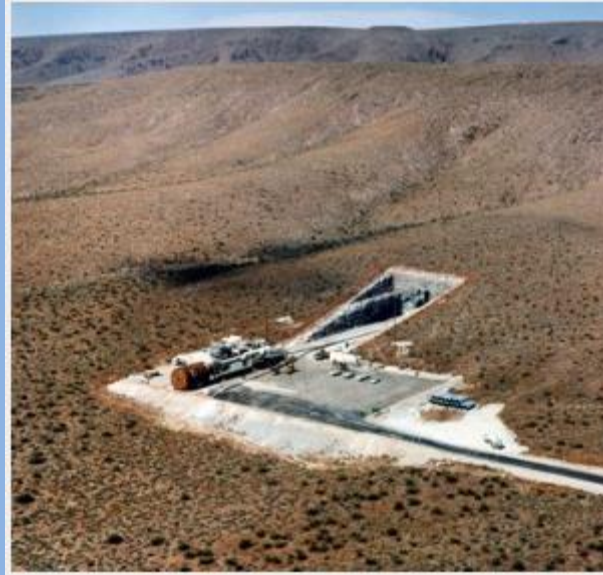
DUMB Deep Underground Military Base Yucca Mountain DUMB Tunnel Entrance
